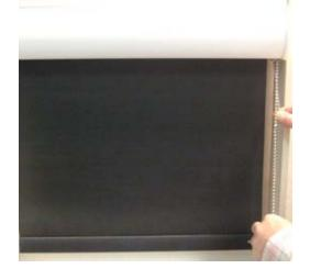
**15.** Remove clear stop bead from chain. Lower shade to desired height. Mark the chain bead on the room side next to clutch. Lower shade a few inches, then place clear stop on the marked bead.
