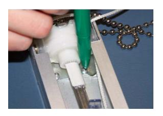
**10.** Using a #11 drill bit (3/16" or .191 in.), drill a hole through the headrail at each marked location. Clear the drilling operation debris from the headrail and pinion rod.
