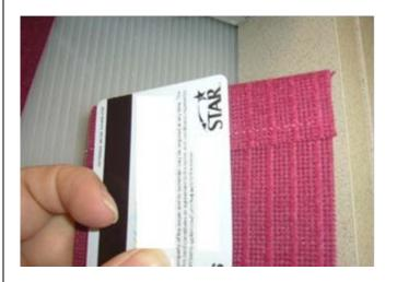
2. Rotate louvers to the open position. Slide a hard plastic card between the louver and the long side of the louver stem. Push the card and louver up toward the top of the stem. This will unseat the louver from the stem.
