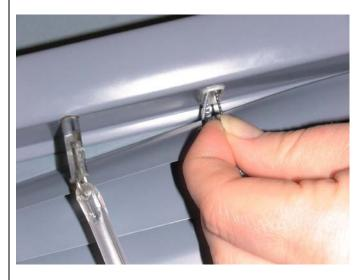
3. Tilt the slats horizontally. Lift and lock the slats in the raised position. Remove the blind from the mounting brackets.
