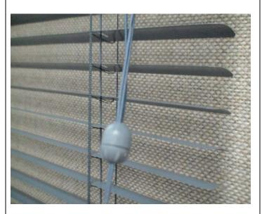
**23.** With the cords even, trim the cords to the desired length but not less than 15". Place a tassel and washer over each cord and secure with a double loop knot.
