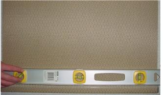
**1.** Check levelness of shade with a carpenter's level and adjust the mounting brackets.
