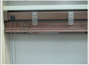
**2.** Remove the blind from the mounting brackets.
