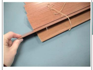
**6.** Using a metal tape measure, measure from the left end of the slat to the middle of the first rout hole. Record this measurement to the nearest 1/16".
