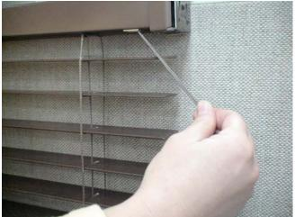
**15.** Adjust the cord stop beads or safety tassel so they are approximately 3" from the bottom of the headrail.
