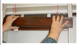
Remove blind from installation brackets using a flat head screwdriver. Place screwdriver under the front lip of all brackets and rotate headrail forward to release.
