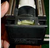
8. Reinstall blind into brackets by slipping the lower lip of the headrail into the mounting bracket. Rotate the front of the rail so that the bracket snaps and catches the front upper lip of the headrail.
