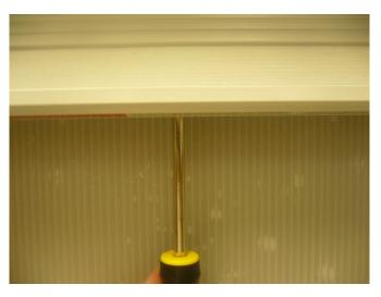
2. Remove screw in top of headrail.
