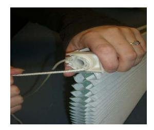
7. Replace shade in the brackets by attaching front of the shade to the front of the brackets and pushing back on the shade until it snaps into place.
