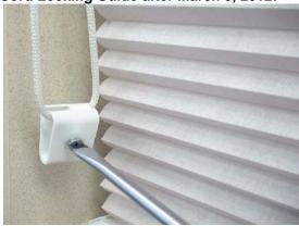
2. Remove shade from installation brackets using a flathead screwdriver. Insert tip of screwdriver between the back of the headrail and the bracket.
