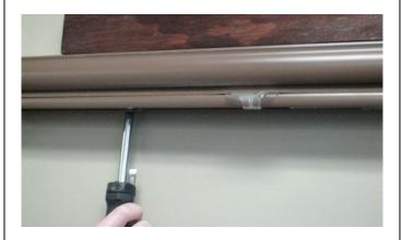
2. Raise and lower shade to see if it works while not in the brackets. If the shade raises and lowers correctly, move the end brackets so they are a minimum of 3" in from each end.
