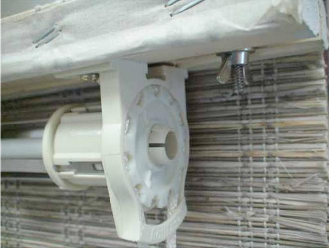
2. Remove screws from base of clutch.
