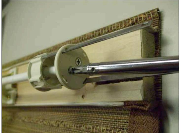
11. Slide the disc to the back of the clutch. Then mount clutch onto headrail.
