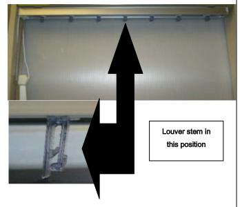
2. Remove louver by pulling down on both the louver and the plastic card at the same time. Lay louver on a clean flat surface. Repeat for all louvers.
