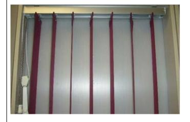
6. To ensure the louvers will rotate correctly, pull the rotation chain several times to turn the stems back and forth, then slide the carriers across the blind by pulling the traverse cord several times. This will assure the cords are moving freely.
