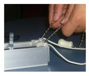
**12.** If stems are moving out of sync, hold rotation chain stationary while turning stem counter clockwise by hand. Stems will turn hard.
