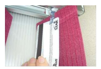
3. Remove the louver by pulling down on both the louver and the plastic card at the same time. Lay the louver on a clean flat surface. Repeat for all louvers.
