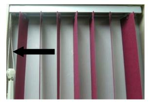
2. Rotate the louvers open and slide a hard plastic card between the louver and the long side of the louver stem. Push the card and the louver up toward the top of the louver stem. This will unseat the louver from the stem.
